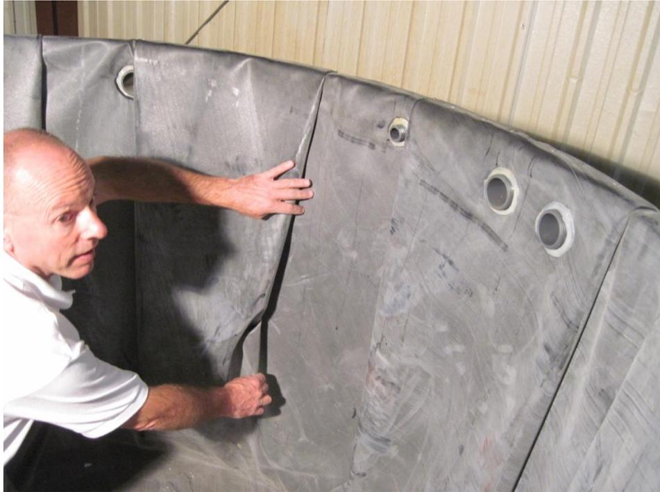
5. Climb inside the tank. Be careful not to damage the liner. Straighten out the pleats of the rubber liner.
