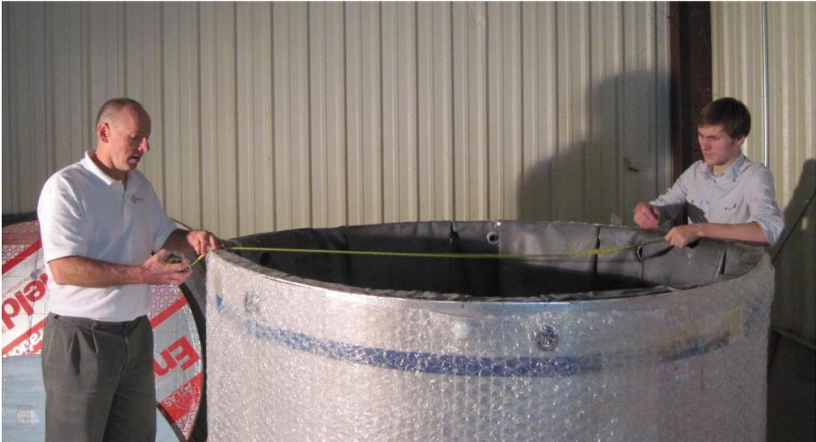
2. Lay the tank bottom on the ground with the blue Styrofoam side facing down.
