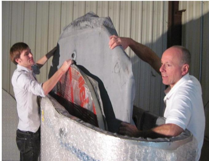
5. Leave the bubble wrap on. Lay the tank down on its side. Remove the crate bottom.
