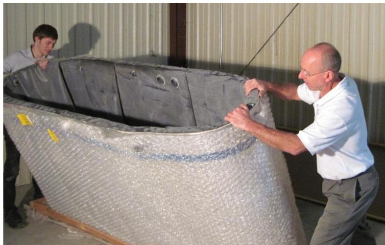
6. With the tank is on its side, push the liner inside the tank. This protects the liner while moving the tank into position.
