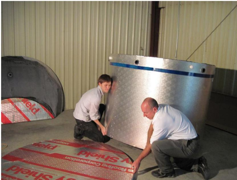
4. Fit the tank shell around the bottom, making sure the shell insulation falls around the edges. It will be a tight fit. Work your way around the shell pulling out and pushing down. **Note:** It may be necessary to get inside the tank, pushing out on the shell to accomplish this.
