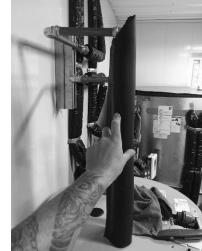
2. Align the insulation along the pipe and cut a hole and/or slit for ball valves, tees, and/or pipe supports
