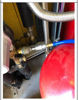
After system is charged turn ball valve in vertical position, close filling port valves and reinstall end caps.
