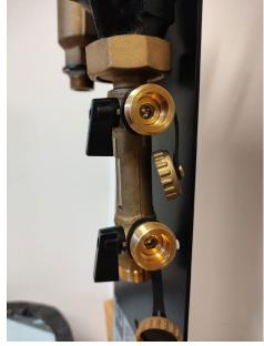
Turn ball valve to horizontal position (preventing glycol from circulating)
