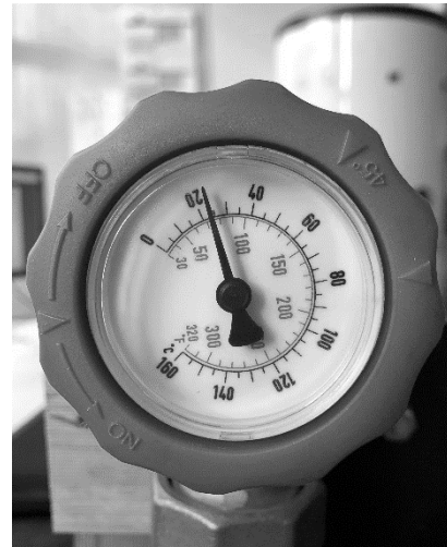
Repair work – ball valve is closed
